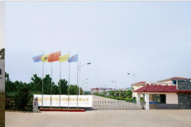
Jiangsu production base
